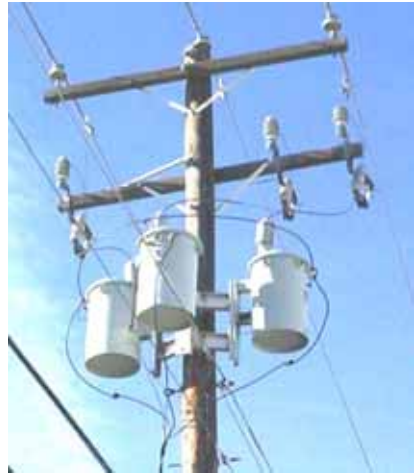
3-Ø Overhead Transformers
